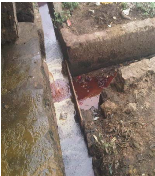
Plate 3. Discharged wastewater into public drains
